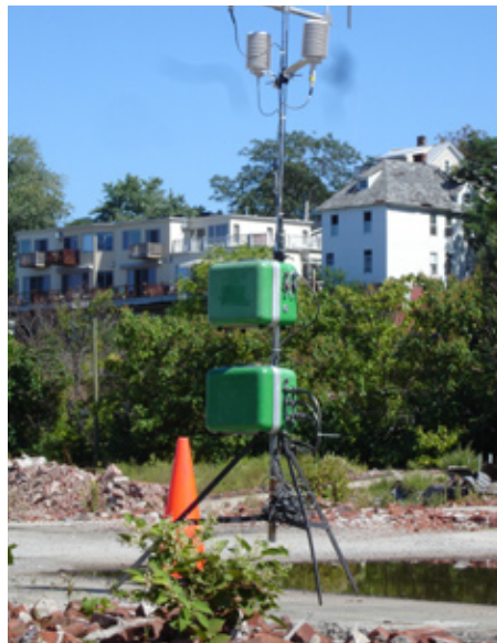
Atlantic Richfield will use real-time air monitoring during demolition.
