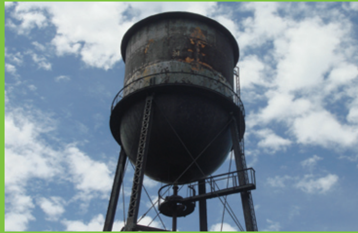
The water tower and the two buildings on the north end of the site are not currently scheduled for demolition.
