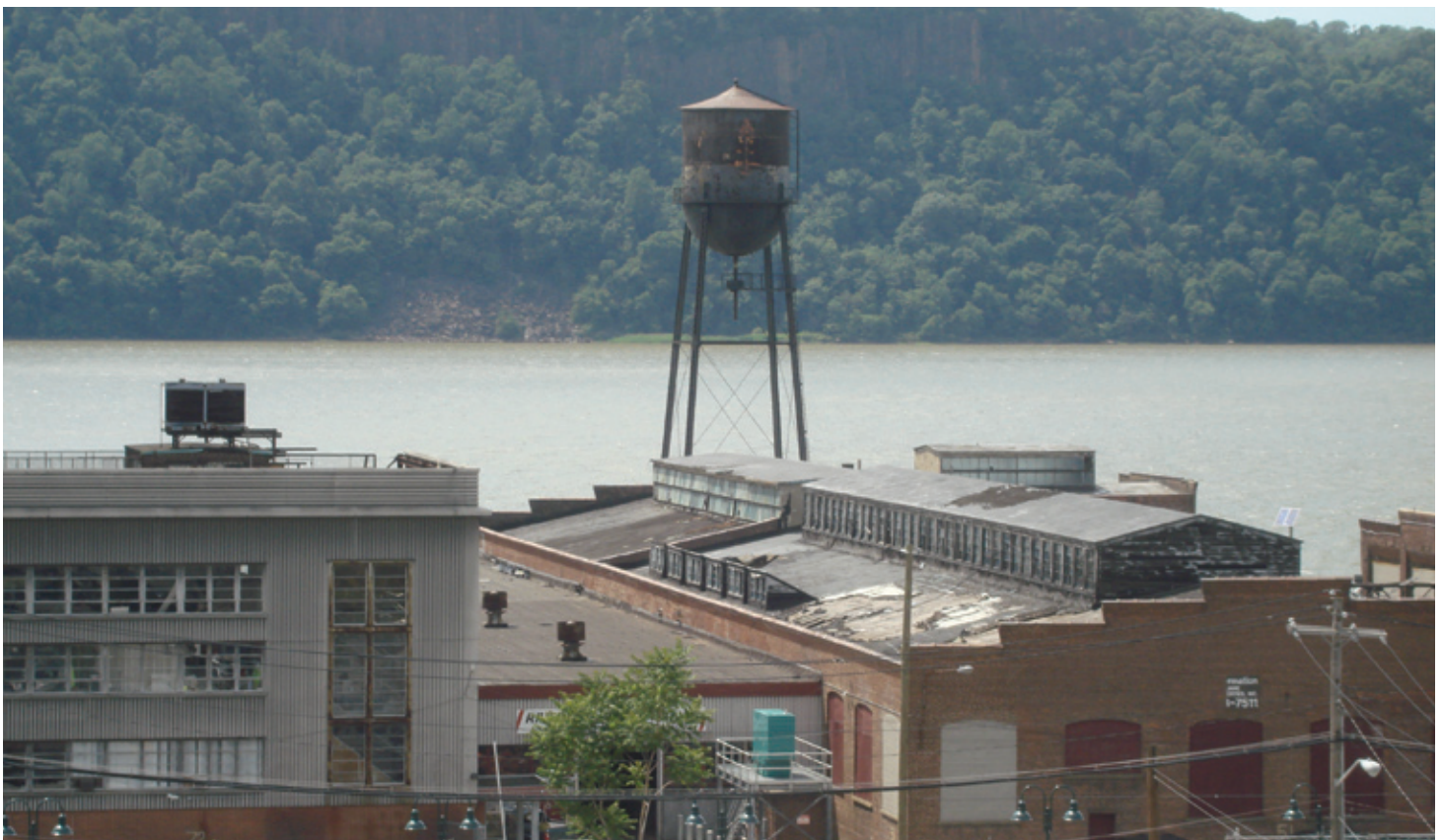
Atlantic Richfield Company will remove 10 structures from the waterfront in preparation for environmental cleanup work.
