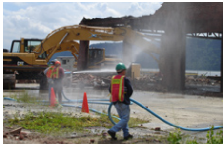
Workers employing dust suppression measures during demolition in 2005.
