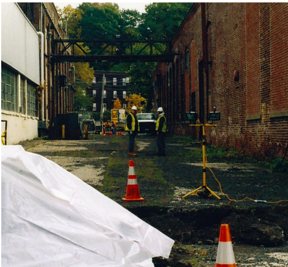
Workers wearing protective gear at an excavation site
