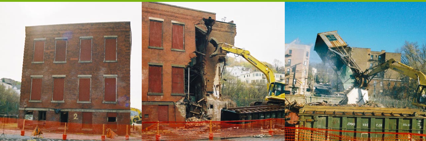
The former administrative building being safely taken down in fall 2004.
